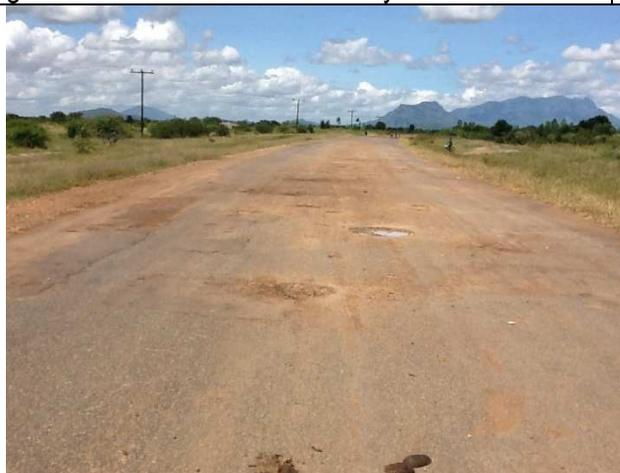
Partially Completed section of Zomba-Jali-Phalombe-Chitakale Road with defects one year after suspension of works due to delayed funding
