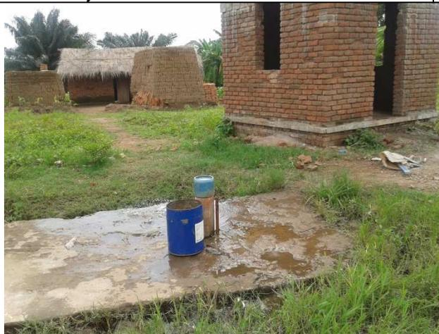
Covered bore waiting to be connected to a pump for NRWB – Songwe Water Supply Project
