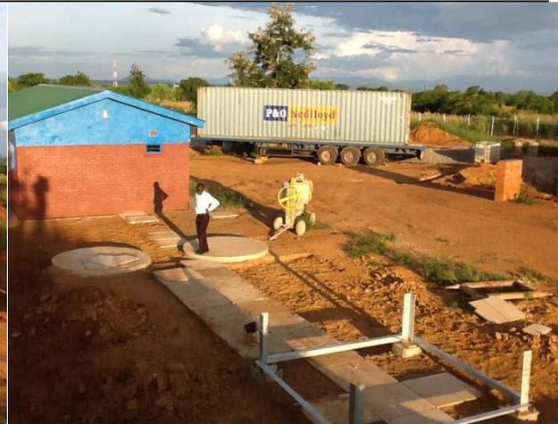
Platform for pressurized filters under construction SRWB – Balaka Water Supply
