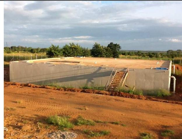
1500 m<sup>3</sup> reinforced concrete tank for SRWB – Balaka Water Supply
