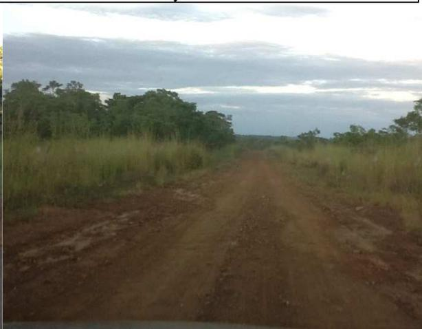
Erosion affecting well-constructed base on Nkhotakota Msulira Road.
