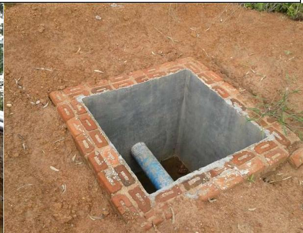
Inspection Chamber on Songani Water Pipeline in Zomba waiting for concrete cover
