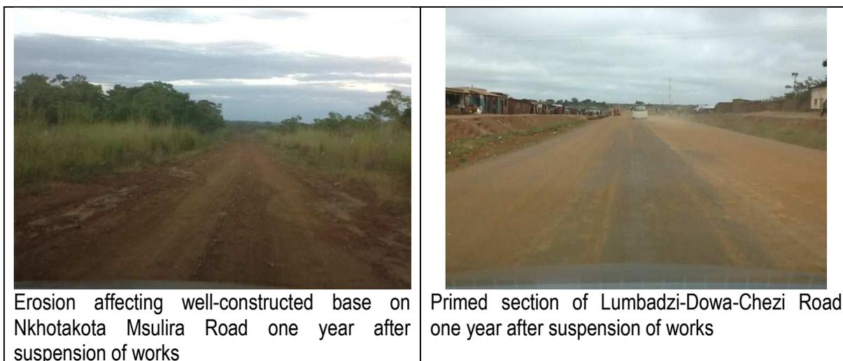
**Figure 3-6 Typical example of the effect of suspension of works**
