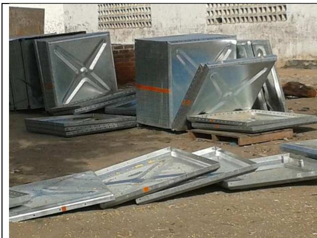
These plates for an elevated tank at Mangochi Water Supply were being hoisted manually.
