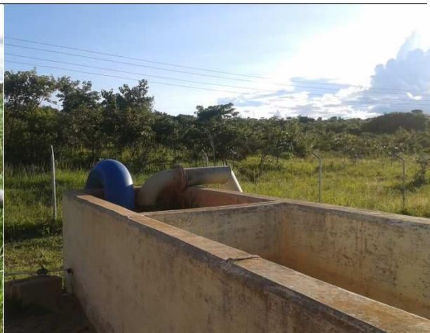
Inlet chamber for 315 mm diameter supply line for NRWB - Mzimba Water Supply Project
