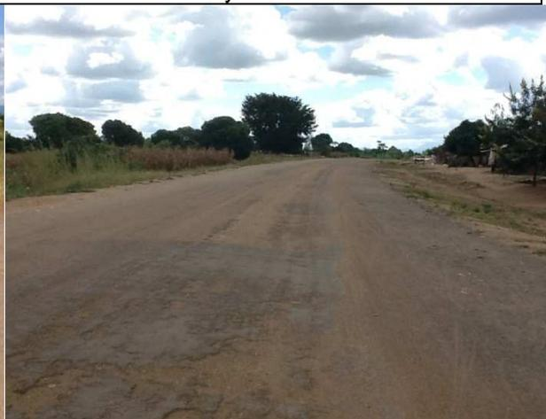
Primed section of Zomba-Jali-Phalombe-Chitakale Road one year after suspension of works due to delayed funding
