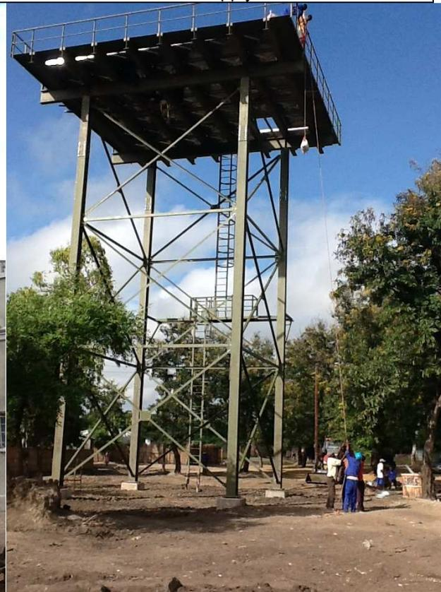
Erection of an elevated steel tank without the use of proper construction equipment. Plates and other units being hoisted manually – SRWB Mangochi Water Supply
