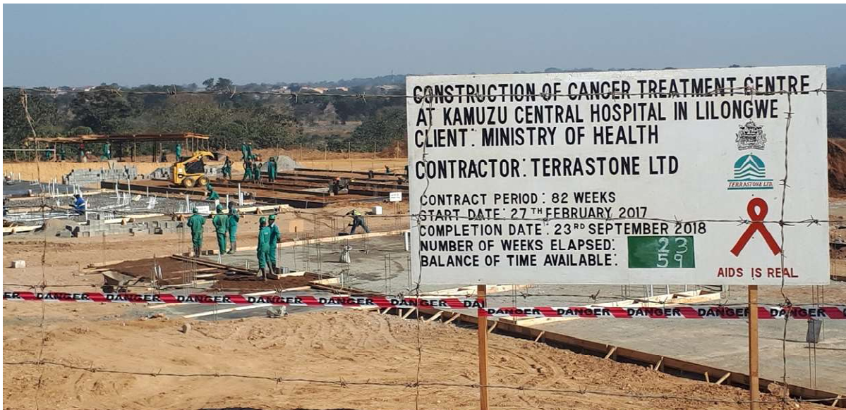
Photo 4.2.2.3 – Foundation works under construction
