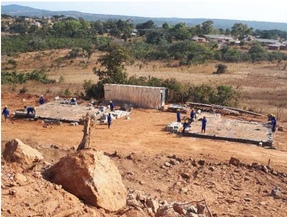
Picture 4.10.3 – Housing foundations at Kazomba Hill
