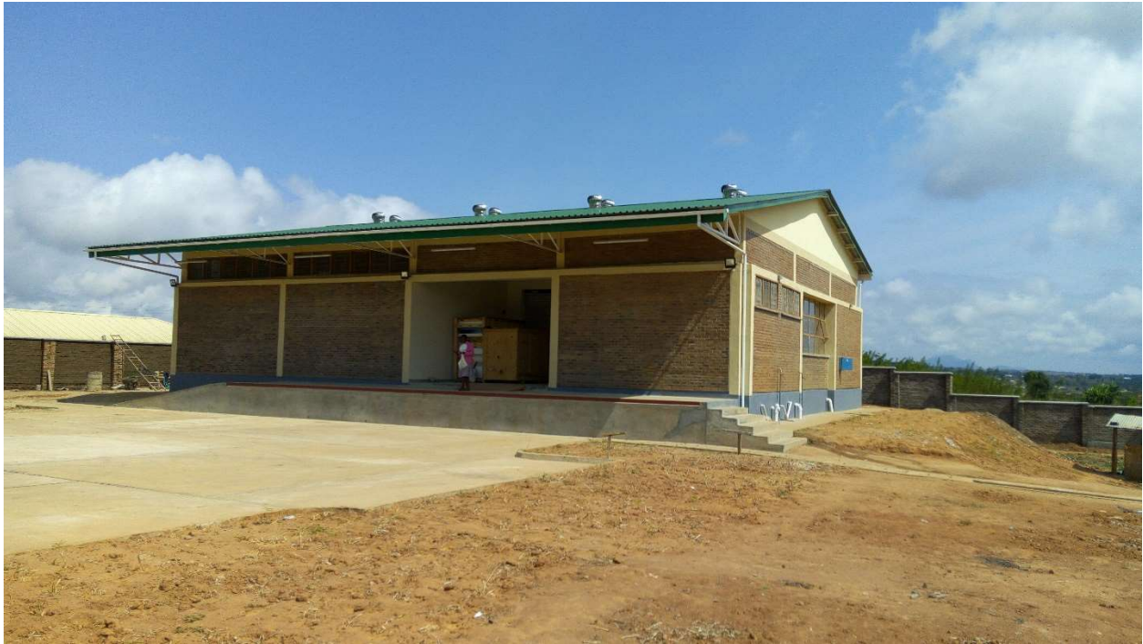
Picture 4.2.3.3 – Picture Showing the Cold Room Facility Externally
