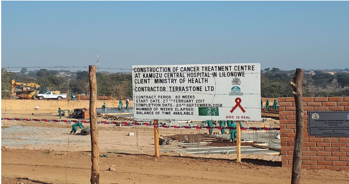
Photo 4.2.2.2 – Project works under construction, Foundation Stone in fore front
