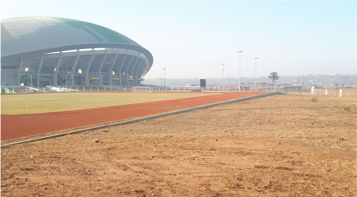
Photo 4.1.2.1 – Showing Landscaped area some shrubs have withered and died
