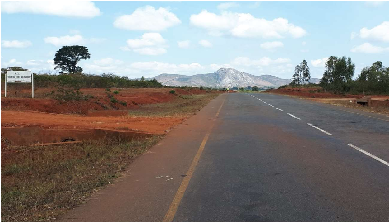
Road showing neat drainage layout; and irregular surfacing
