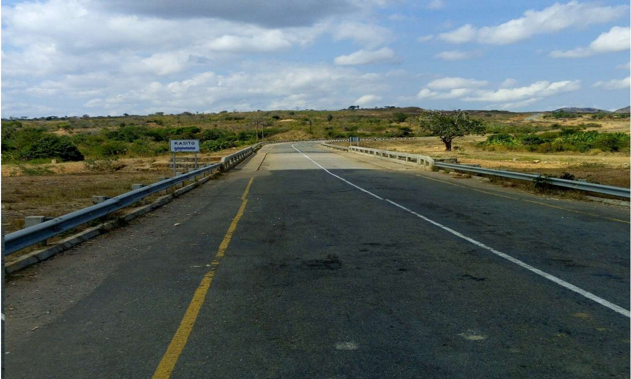
Road Section at Kasito Bridge
