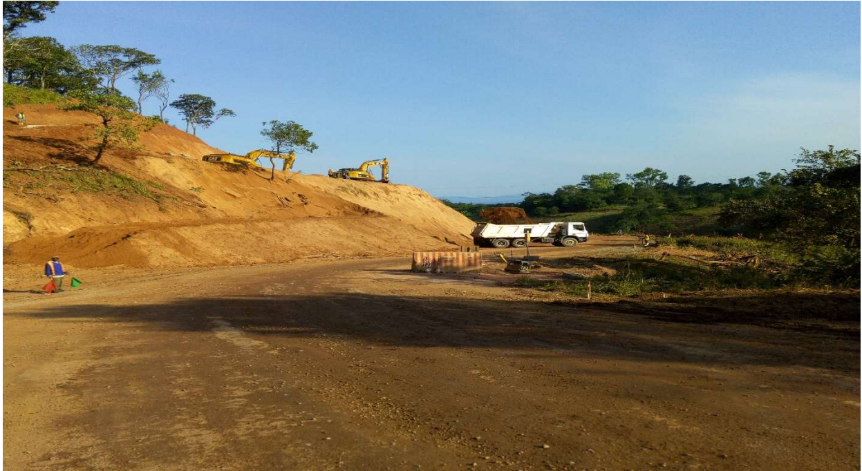
Picture 4.4.4.1 – Benching Slope Protection against Earthworks Collapse
