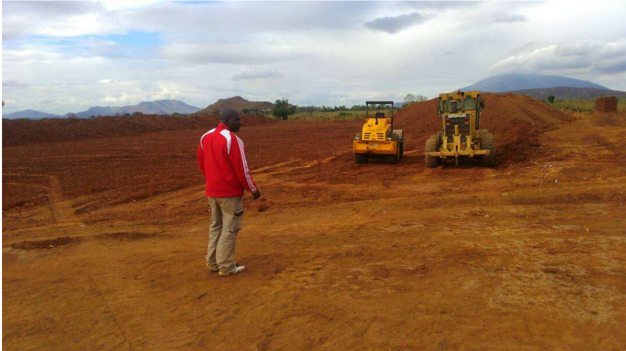
Photo 4.2.1.2 – Site Clearance Works in Progress
