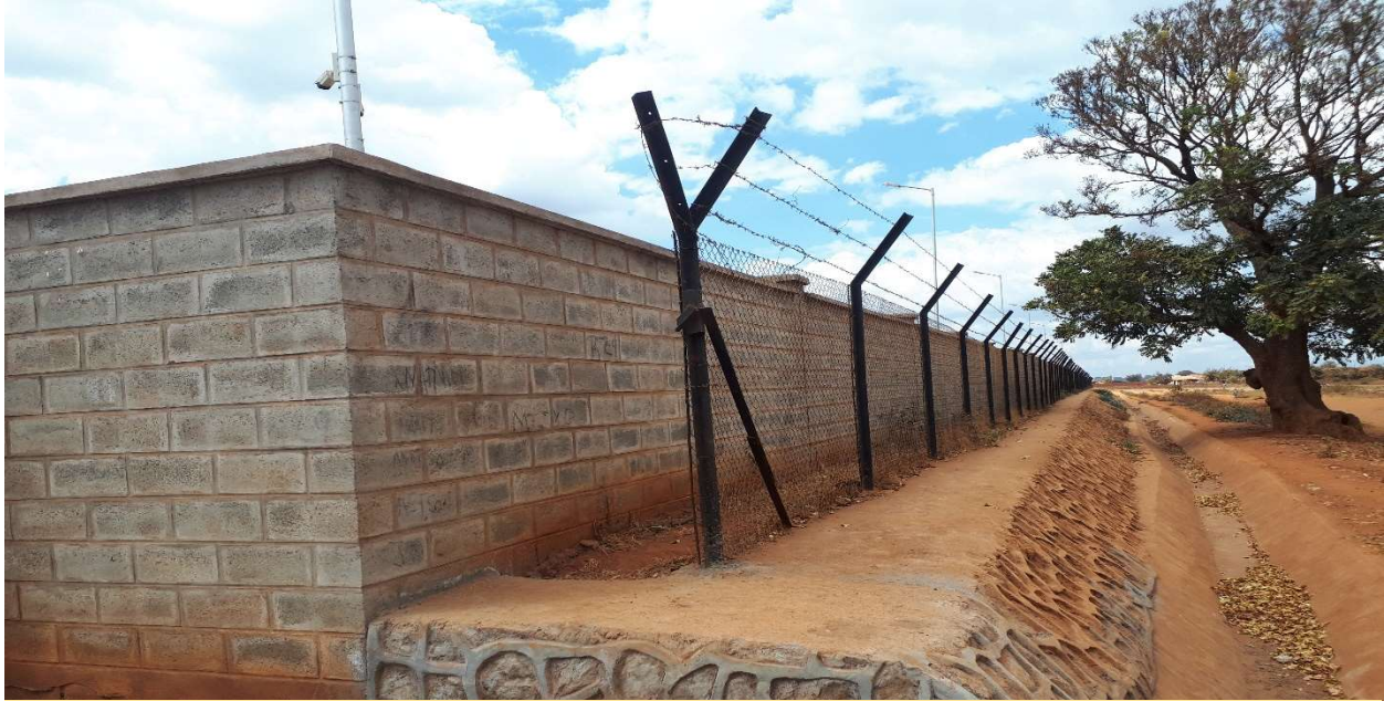
Photo 4.3.2 – New Fence at NOCMA Yard
