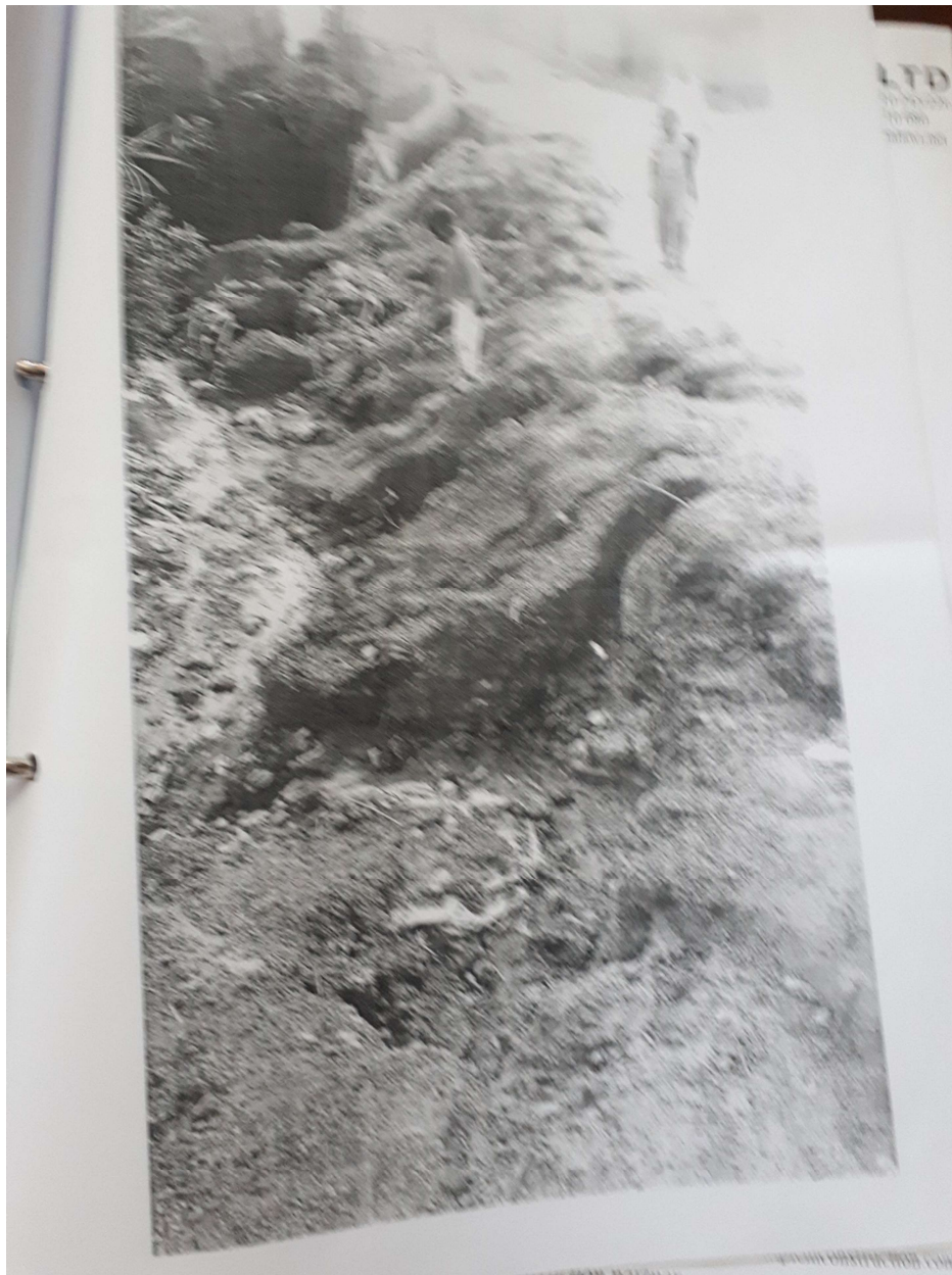
Picture 4.11.1 – Extent of damage due to rain
